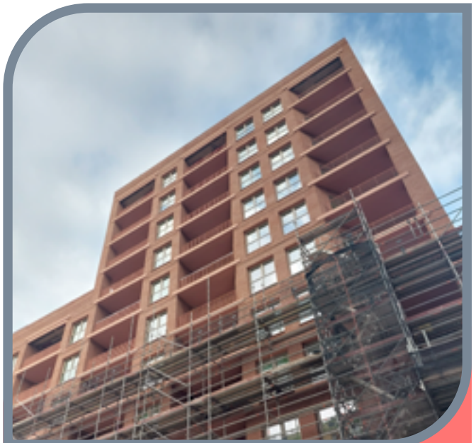
Continuing to build 332 homes, 72% of which are affordable tenures
