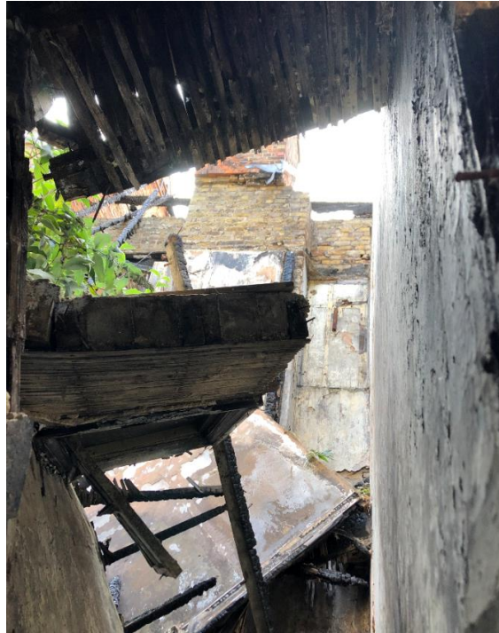
Photo 19 - Apartment 12 view of second floor and roof
