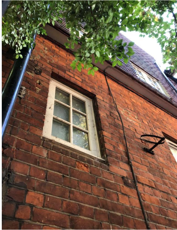
Photo 21 - North side elevation of Main Building
