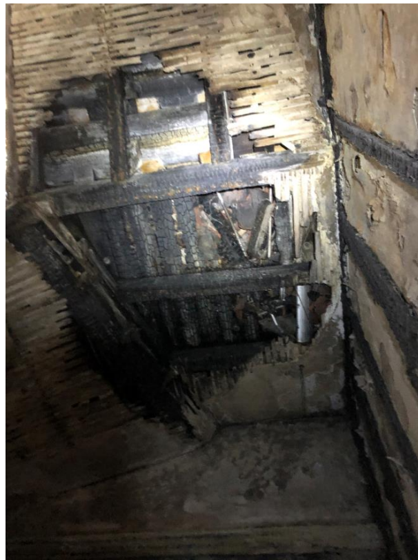
Photo 6 - Apartment 1 bedroom 3 cupboard underside of stair
