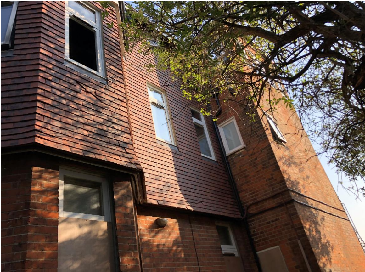
Photo 25 - South side elevation of main building
