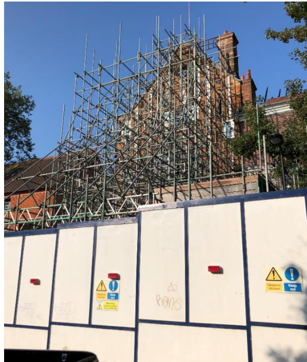
Photo 20 - Front façade gable and scaffold
