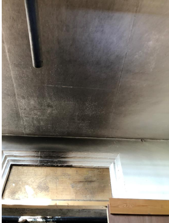
Photo 7 - Main entrance porch
