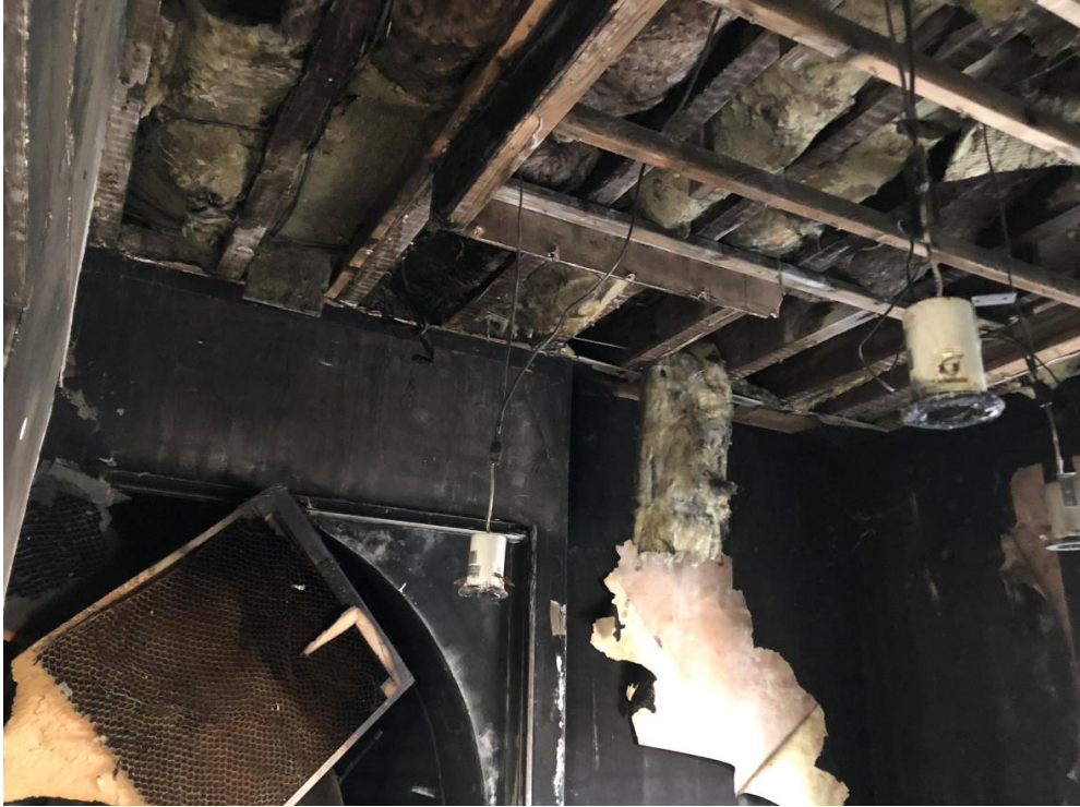
Photo 30 - Timber joists at second floor above apartment 8
