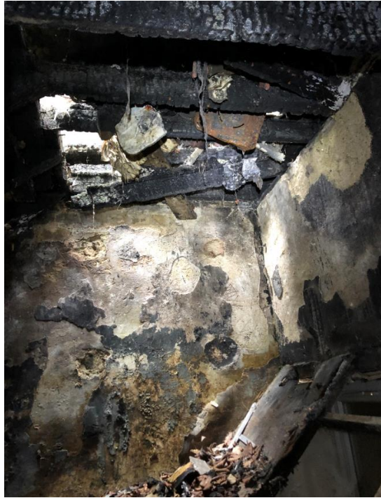
Photo 15 - Stair from ground to first floor underside of half landing
