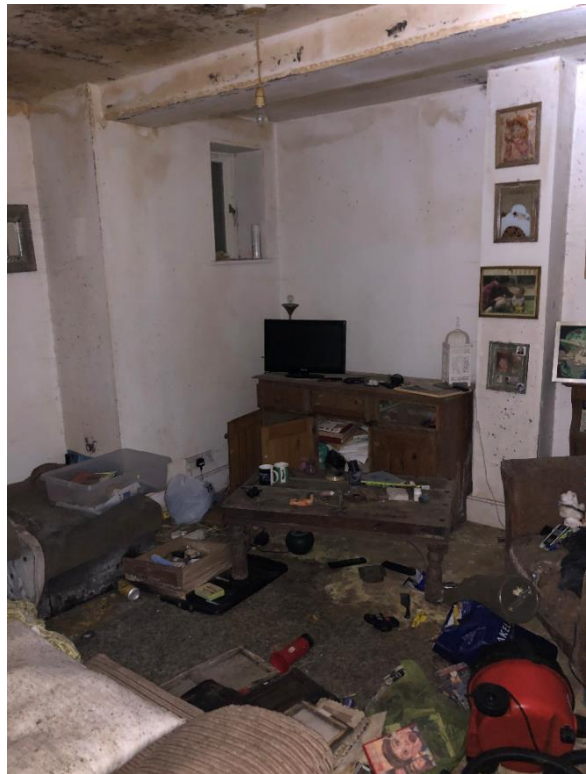
Photo 4 - Apartment 1 living room
