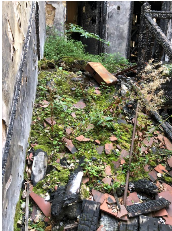
Photo 16 - Stair from ground floor to first floor
