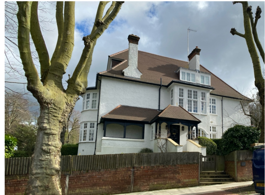
Property in Rosecroft Avenue with bay and dormer windows and open porch. Mature street trees are part of the character.
