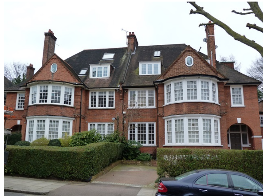
Grade II Listed Nos. 25 and 26 Heath Drive
