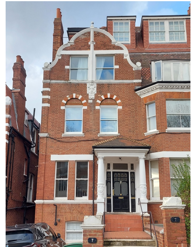
Distinctive Dutch gable feature that is exhibited on many Positively contributing buildings in the Area
