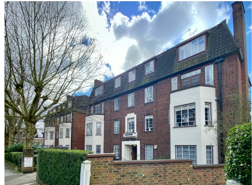
Bracknell Gardens Mansion Block in Bracknell Gardens (with frontage also to Frogna Lane). This has mansard roofs and bay and dormer windows, in common with older properties, but with horizontal emphasis window panes. Note also the stepped door surround.
