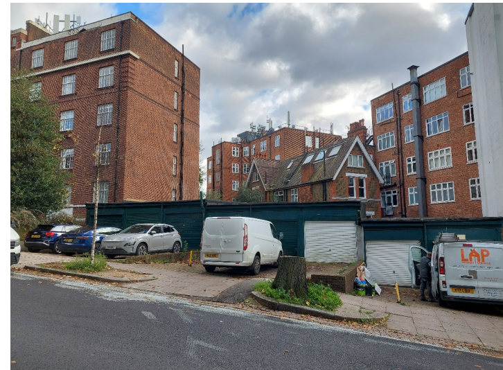
Street frontage garages create harm to the character and appearance of the street.
