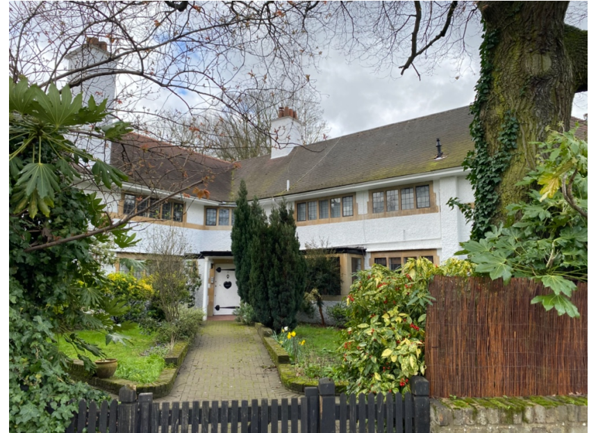
Annesley Lodge at the corner of Platt's Lane and Kidderpore Avenue, designed by Voysey.
