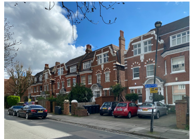
Properties in Frogna Lane have group value with their Dutch Gables and arched window heads. Note the harm caused by the loss of front boundary and garden to create hard surfaced front parking court.
