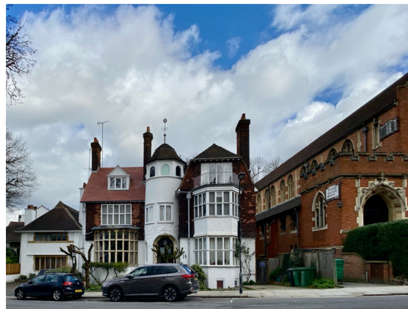
Kidderpore Avenue and Kidderpore Gardens are architecturally diverse. The Northwest end of Kidderpore Avenue includes a group of buildings of exceptional quality.
