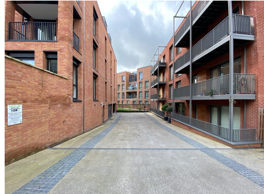
This large-scale development off Kidderpore Avenue introduces a more urban character and makes little concession to the verdant landscaped character of the Conservation Area. Architecturally, it represents a good standard, but the urban form and extensive hard surfaced areas are harmful.
