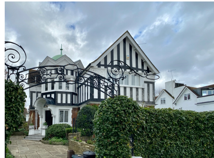
Showing the dwellings along Kidderpore Gardens from the junction with Kidderpore Avenue
