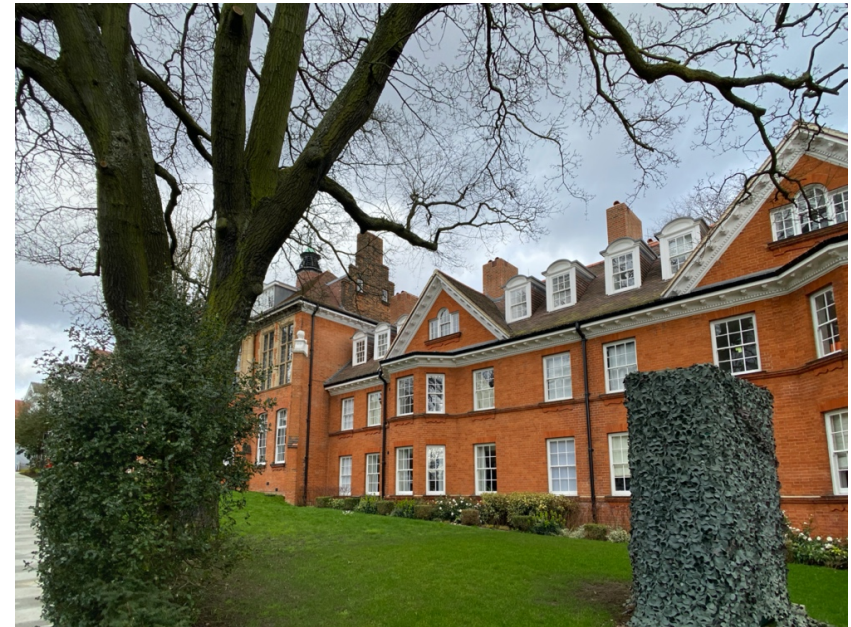
Part of Kings College in Kidderpore Avenue. This comprises large institutional buildings in different styles and from different periods, including Queen Anne Revival.
