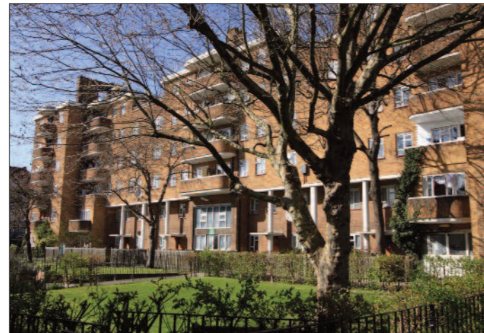
▲ Willingham Close Estate, is composed of three blocks. Willingham was built first as mews properties and took a direct hit from a bomb. It was rebuilt, followed by Rosemary and Margaret House. The Estate was designed and built by a St Pancras in-house team. It was opened in 1952. Cecil Rhodes House in Camden Town was built using the same basic design. One of the residents says, "The Estate is a wonderful example of council-built buildings. The layout, either by design or luck, has produced a great community spirit among us all and I am a great believer that buildings do affect how people live."
