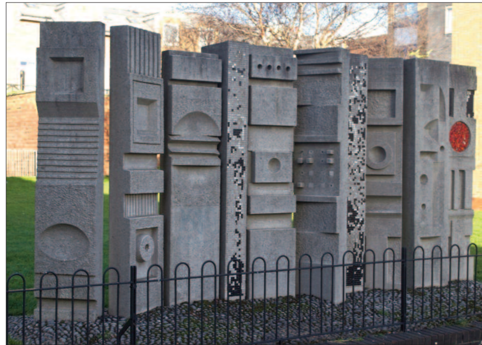
◀ Concrete and mosaic brutalist sculpture situated on the Raglan Estate, Raglan Street. This is unusual example of 1960's civic art, in need of reconditioning of mosaics.
