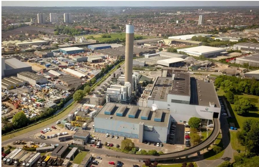
Figure 4.7 - Energy from Waste heat networks are centred around using heat that is produced by the process of waste incineration (above the North London Edmonton incinerator) distributing that heat to homes close to it or much further (Photograph: pxl.store/Alamy)
