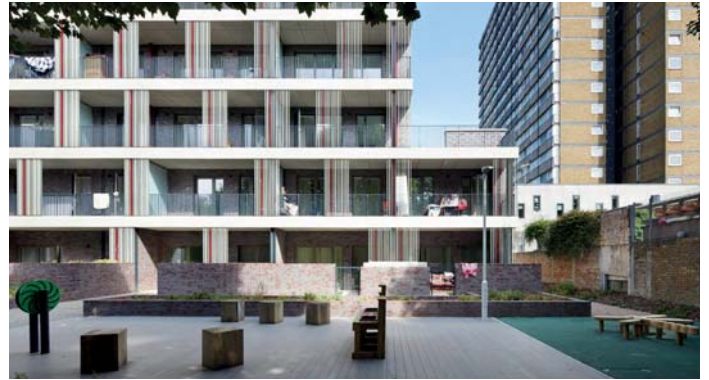
Rear view of Block A - now called Flats 1-38, 14-16 Wrotham Road - which comprises 38 council homes and completed in April 2018. Recently, the building won two awards in the New London Architecture Awards 2019: Overall Winner and Sustainability Prize
