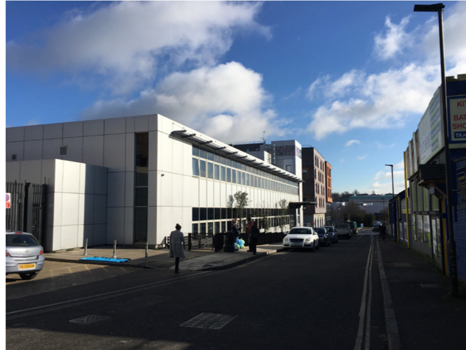
Existing building (looking east)
