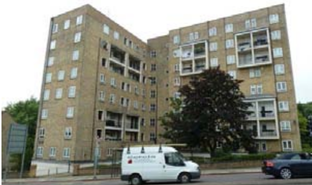
Substantial blocks in Swiss Cottage
